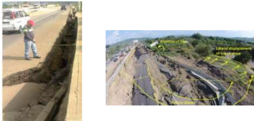
Figure 2.3. Road displacement and embankment slope failure in Manta, Ecuador 2016.
