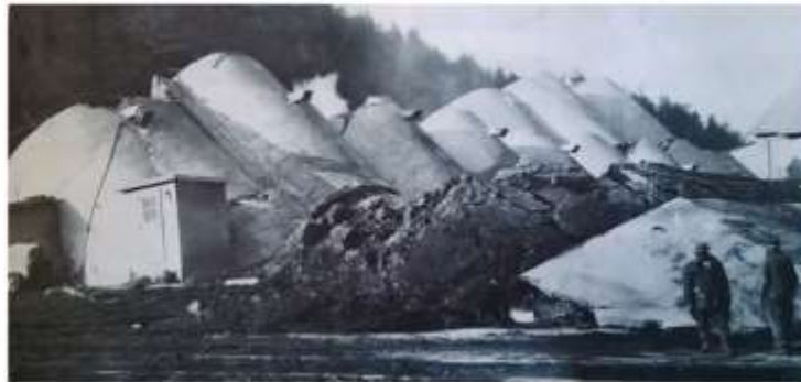
Figure 2.4. Loss of bearing capacity in a silo foundation structure due liquefaction (1951). (McManus, 2016)
